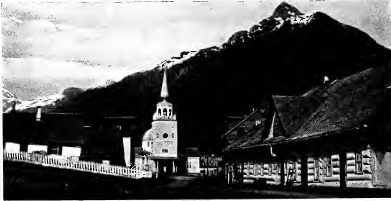
The Russian warehouse at the head of the wharf at Sitka was built of huge logs, the bottom rounds being over three feet in diameter.
